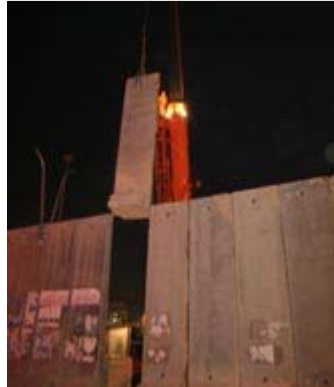
The last brick in the wall. Closing the remaining gaps in the wall near A-Ram. Photo: Roberto Costonovo
